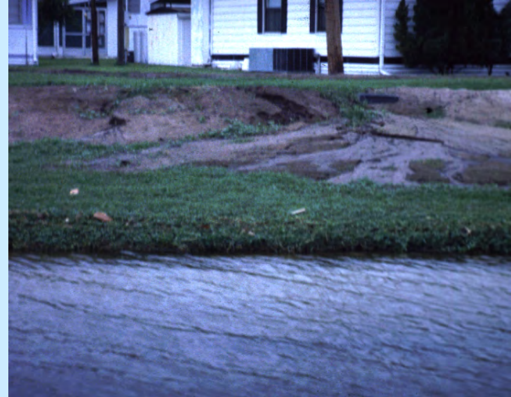
Failing septic tank
